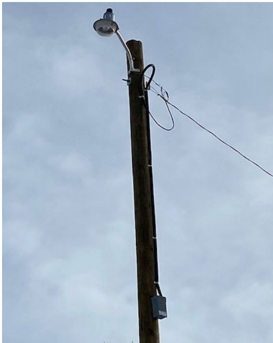
Figure 4: Christmas light servicing on wood poles
